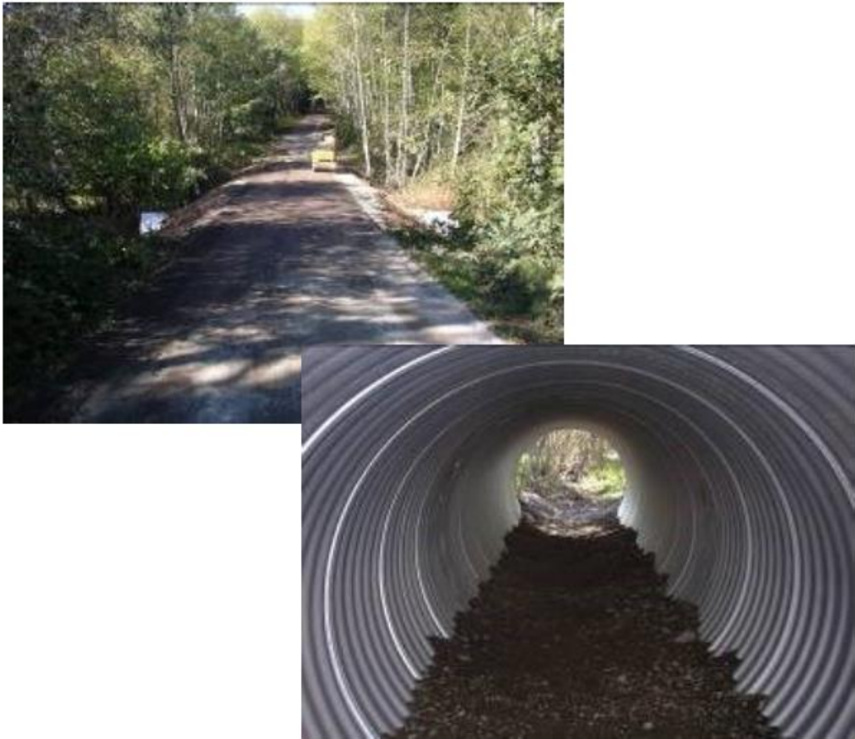
Figure 3 – Post-construction photos for 7-foot diameter culvert replacement under Buttram Lane (2006)
