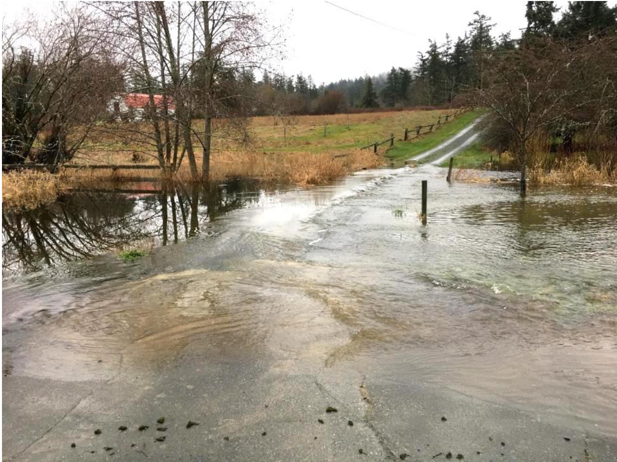
Photo 7 – Shallow flooding over private driveway upstream of Buttram Lane (February 2020)
